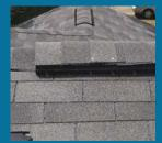
Most attics are designed to be vented. Air moving through the attic keeps the house healthy and utility bills down. One way to move hot air out of an attic is through **ridge vents**. These are located at the peak of the roof.
