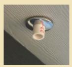
The **secondary A/C drain** is located above a window. If water backs up at the system in the attic it will drain out of this pipe. If this happens, call for service immediately.
