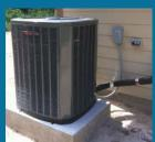
The A/C unit on the outside (**the condensing unit**) is secured to a concrete pad. This pad should always be higher than the grade around it. Also, do not allow plants to grow close to it nor construct anything around it that will hinder air
