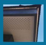
In order to vent air out the ridge vent or air hawks, you must have **soffit vents** to let cool air in. The overhang (soffit) is designed to allow air in and then rise up through the attic as it gets warmer. It is then vented out.
