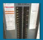
**Electric panels** may be located in the garage, inside the home, or on the exterior. Each breaker is labeled. When resetting a breaker, first push it all the way to the "off" position and then reset it. To turn off power to the entire house, simply flip the main breaker to the "off" position.
