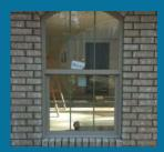
Before closing, a high quality **caulk** was placed around the windows at masonry work. This should be checked periodically and maintained as needed.
