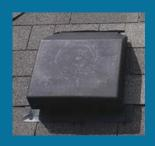
Another way to vent air out of the attic is through the use of "air hawks." These square vents are placed in numerous areas around the roof.
