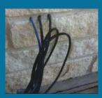
The connection points for your phone and TV wires are usually close to the electrical service. The blue wire is for phone service and the black wires are for TV service. These wires will run from the outside to a structured wiring box located inside the house.
