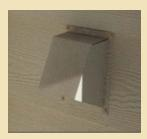
If your home has a fireplace, it requires **combustion air** from the outside to burn gas or wood. A small air duct has been run from the outside to the fireplace for this purpose.
