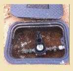
If your home is hooked up to a public water supply, there will be a **water meter** in an underground box in your yard. One or two shutoff valves may be located here to allow the water to the house to be shut off.
