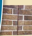
Brick veneer and stone walls expand and contract based on the temperature outside. In order to control cracking, **expansion joints** have been designed into the wall to allow for movement. A silicone sealer has been added and should be maintained as required.
