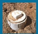
Occasionally a plumber may have to unclog a pipe. He'll do this by using one of the **clean outs** installed in the system. The main house clean out and some smaller clean outs are visible around the exterior of the home.
