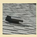
Depending on the design of the home, sometimes a **dryer vent** goes out through the roof. When that is done, a device similar to this may be visible on the roof from the ground.
