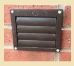
A **dryer vent** usually goes straight out of a wall. When this is done, a simple cover like this is commonly placed over it. Check it periodically to make sure it is not blocked by lint or even a bird's nest.
