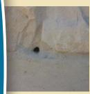
Similar to the **weep holes** described above, stone walls require similar devices. Round holes will be seen at the base of stone walls to allow water to drain out and for air to circulate in.
