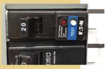
The National Electric Code requires numerous safety devices to be installed in new homes. The purpose of this handout is to point out two of these important features. Ground Fault Circuit Interrupters (GFCI) and Arc-Fault Circuit Interrupters (AFCI) are designed to protect from certain electrical hazards.
