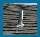
The Plumbing Code requires the system to be properly vented. **Plumbing vents** are a series of pipes that run up and out through the roof.
