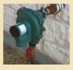
A home that has propane gas service will have a tank located in the yard. From there, a gas line will be run to the house. A shutoff valve is located just before the **regulator**. The metal gas lines may be bonded at this point as evidenced by a clamp and a copper wire.
