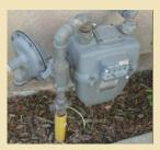
If your home has natural gas provided to it, there will be a **gas meter** located at or near the house. The metal gas lines may be bonded at this point as evidenced by a clamp and a copper wire. If you smell gas, call your gas provider.
