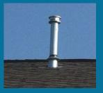
Gas and propane water heaters are required to be vented to the outside. This will be done with a metal vent pipe. The small disc toward the bottom ("storm collar") should be properly sealed to ensure water tightness.
