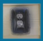
**GFCIs** on the outside are usually located at exterior doors, by the A/C unit, on balconies and porches, or on the outside of a garage. The one shown to the left (in a protective box) is common when it is exposed to the weather.
